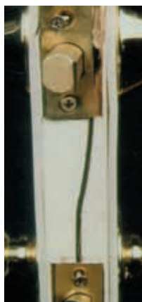
A wood edge steel door cracks under force of one hit of a 100lb. test weight.
