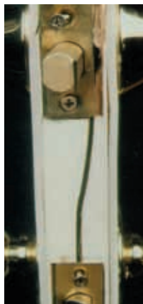
A wood edge steel door cracks under force of one hit of a 100lb. test weight.
